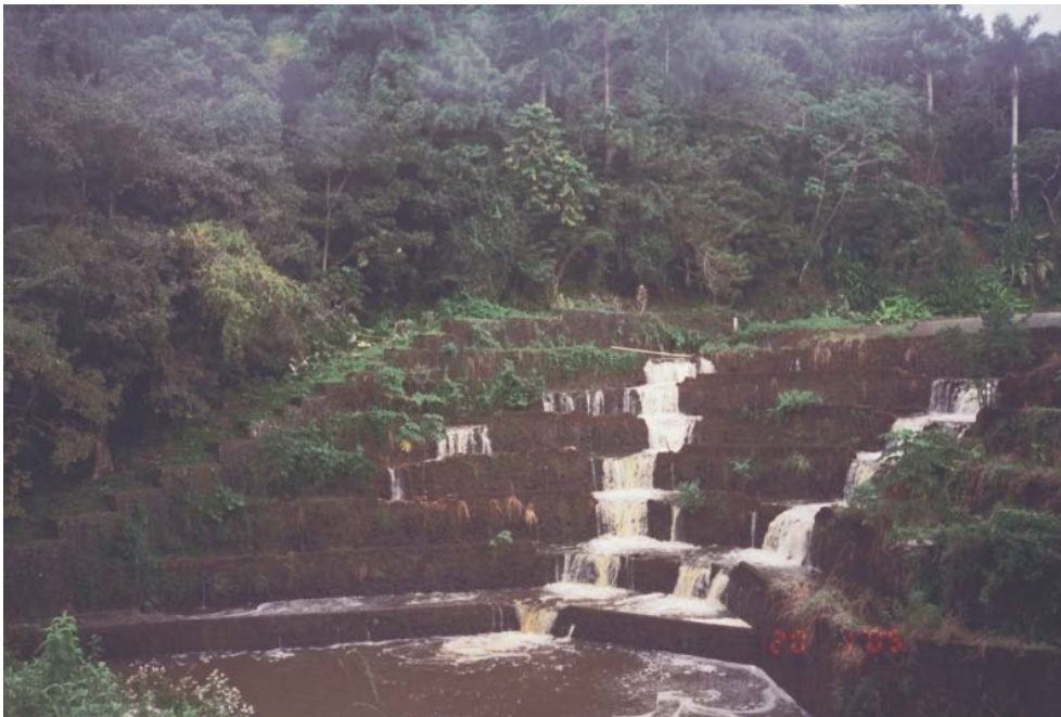
Figure 1 – Masonry spillway in need of rehabilitation
